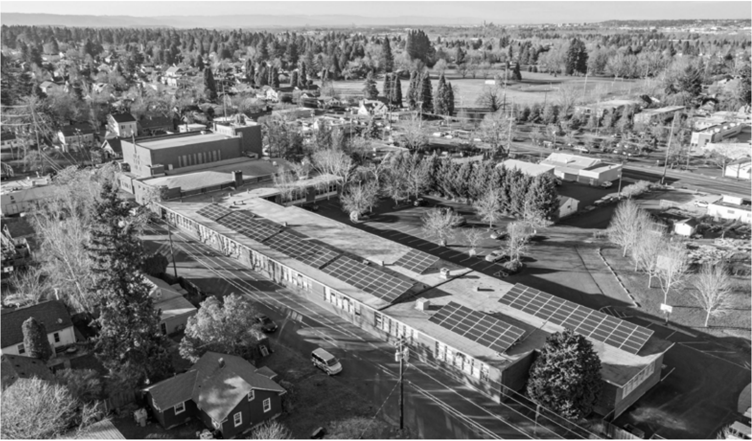
Facing northwest, this photo displays the new solar panels on St. Charles Catholic Church's classroom building. Energy savings are estimated at $7,481 per year, which helps the parish focus more resources on community work. Photo courtesy of Neil Kelly Company
