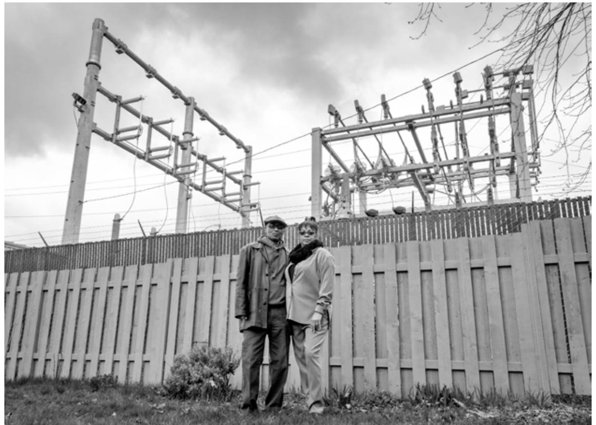
Michael and Linda Kelsaw have a new view from their back yard. Pacific Power’s Kennedy Substation came out of mothballs beginning last autumn with an expansion plan that caught neighbors by surprise. Additionally, a mix of new wood and steel power poles will replace old ones on 41st Avenue. Photo by Chris Baker
