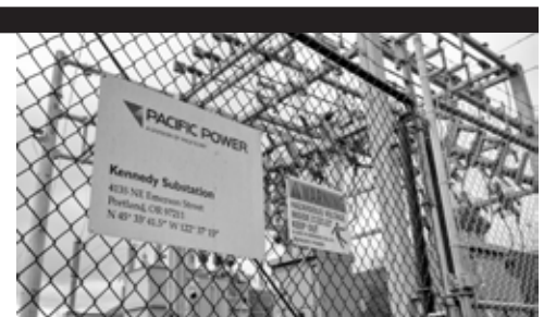
NEIGHBORS EXPRESS DISSENT Residents are surprised, concerned about substation expansion.
