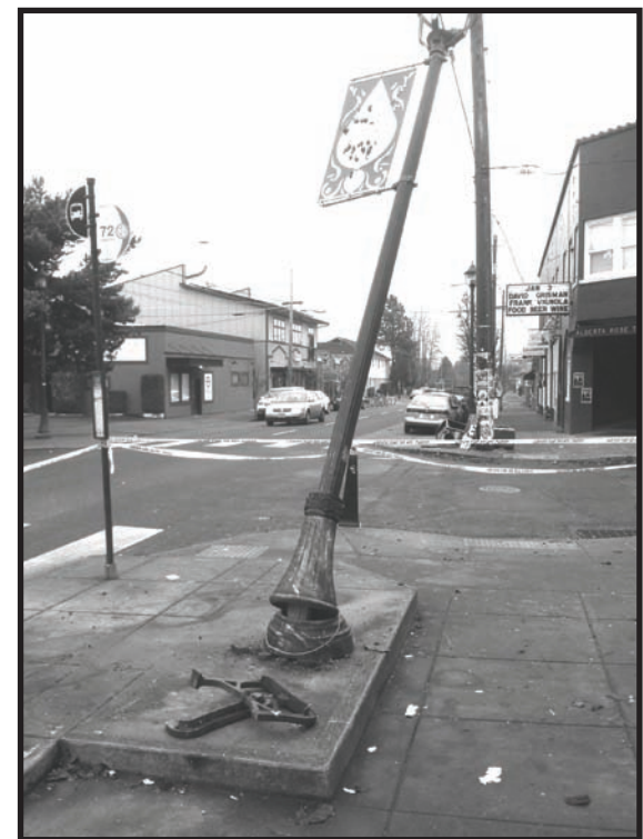
Defying gravity. An accident that destroyed the street furniture left the lamp post askew. The City replaced it and re-hung the metal banner, the next day.
