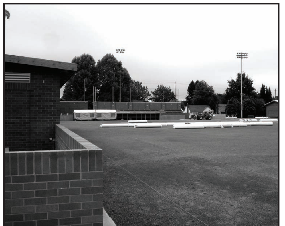
Getting ready to roll out the turf. Looking toward the infield from the corner of right field.
