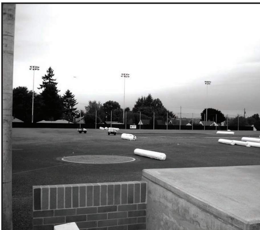
Looking toward left field from behind the first base dugout. The circle is where the pitcher's mound will be built.
